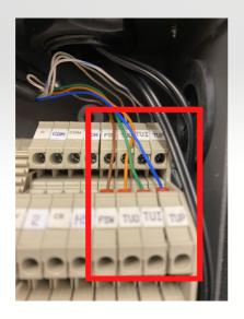
These are the connections for the premade cable that goes between the heat pump and indoor unit
