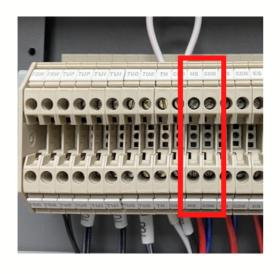
For external controls your call for heat should go into "hs" and "com" The neutral wire from your heating controls should be connected into com.
