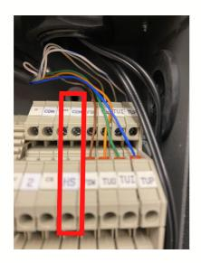
For external controls your call for heat should go into hs and com (neutral into com).
