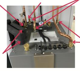
Two 1" male connections middle and high temp hot outlet
